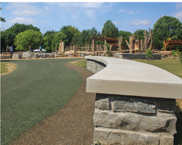
FLEXI-PAVE AND STONE SEAT WALL
